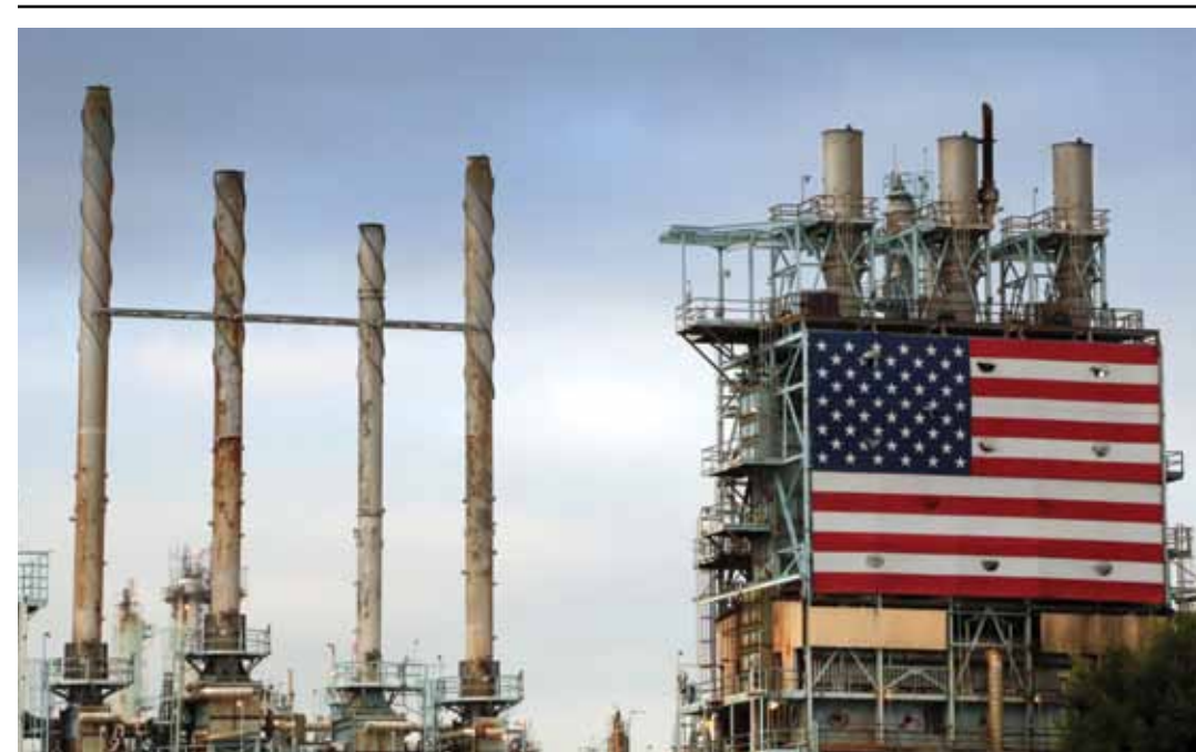
An oil refinery in California
